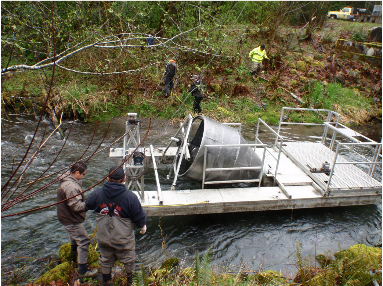
Figure 4. Installing Little River screw trap, spring 2014.
